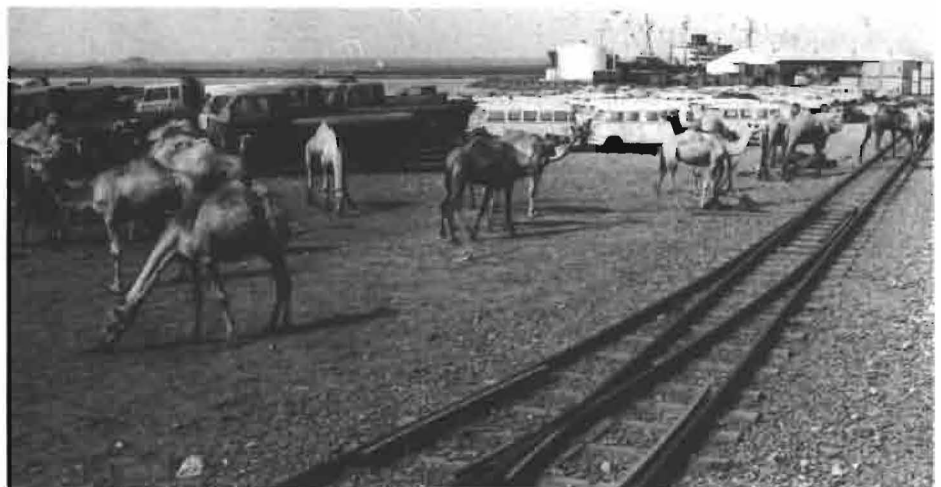
The Djibouti railhead
