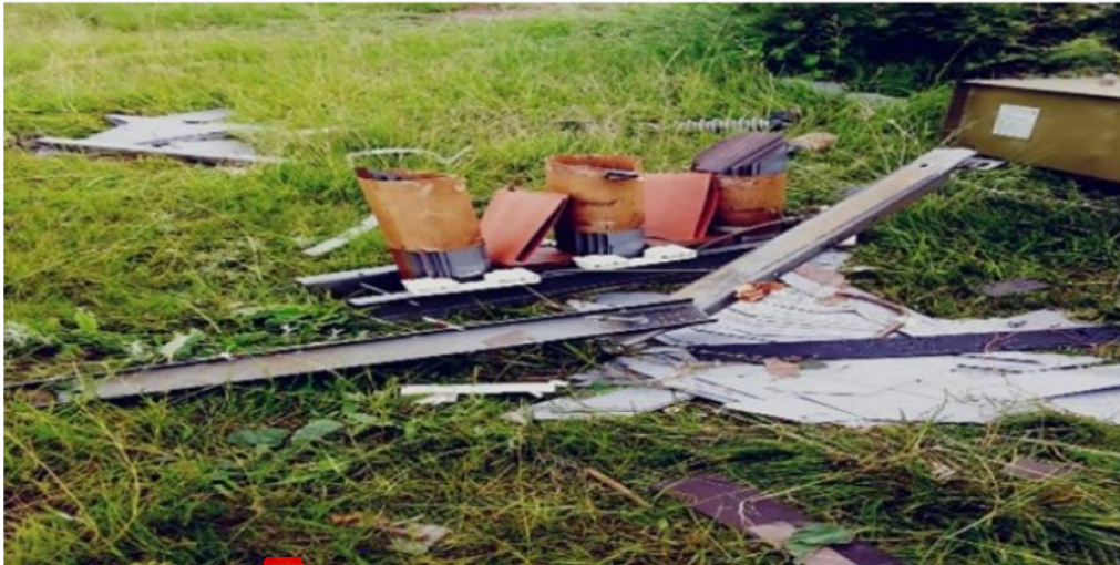
25 Figure 2: The ugly face of water and sanitation infrastructure vandalism
