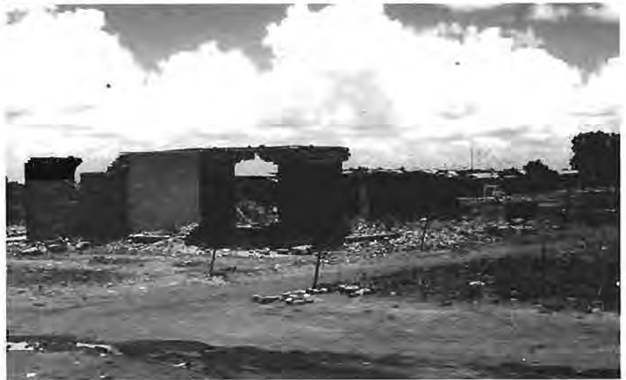
Demolished house in Botshabelo.
