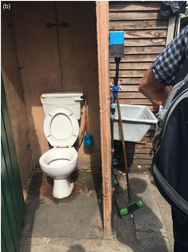
Figure 6b. Shared backyard toilet facility.
