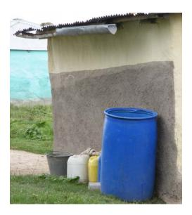
Rainwater harvesting with water barrels is common. Although it is not particularly efficient as rainwater is often blown from the open barrel it is relatively cheap.
