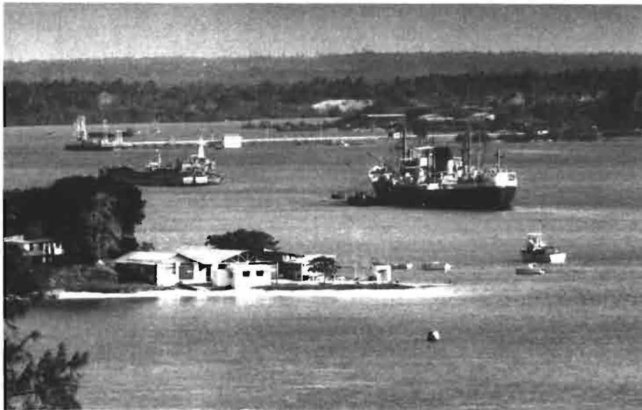
Dar es Salaam harbour. The Chinese have been building extensions at the far end
