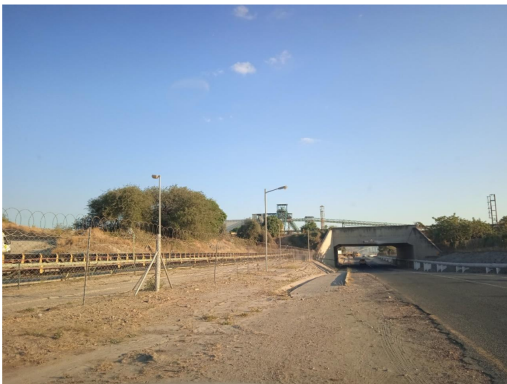
Figure 3: Foskor mining infrastructure
