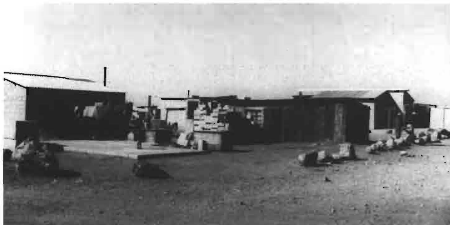
Self-help housing. Living in a shack while the house is being built
