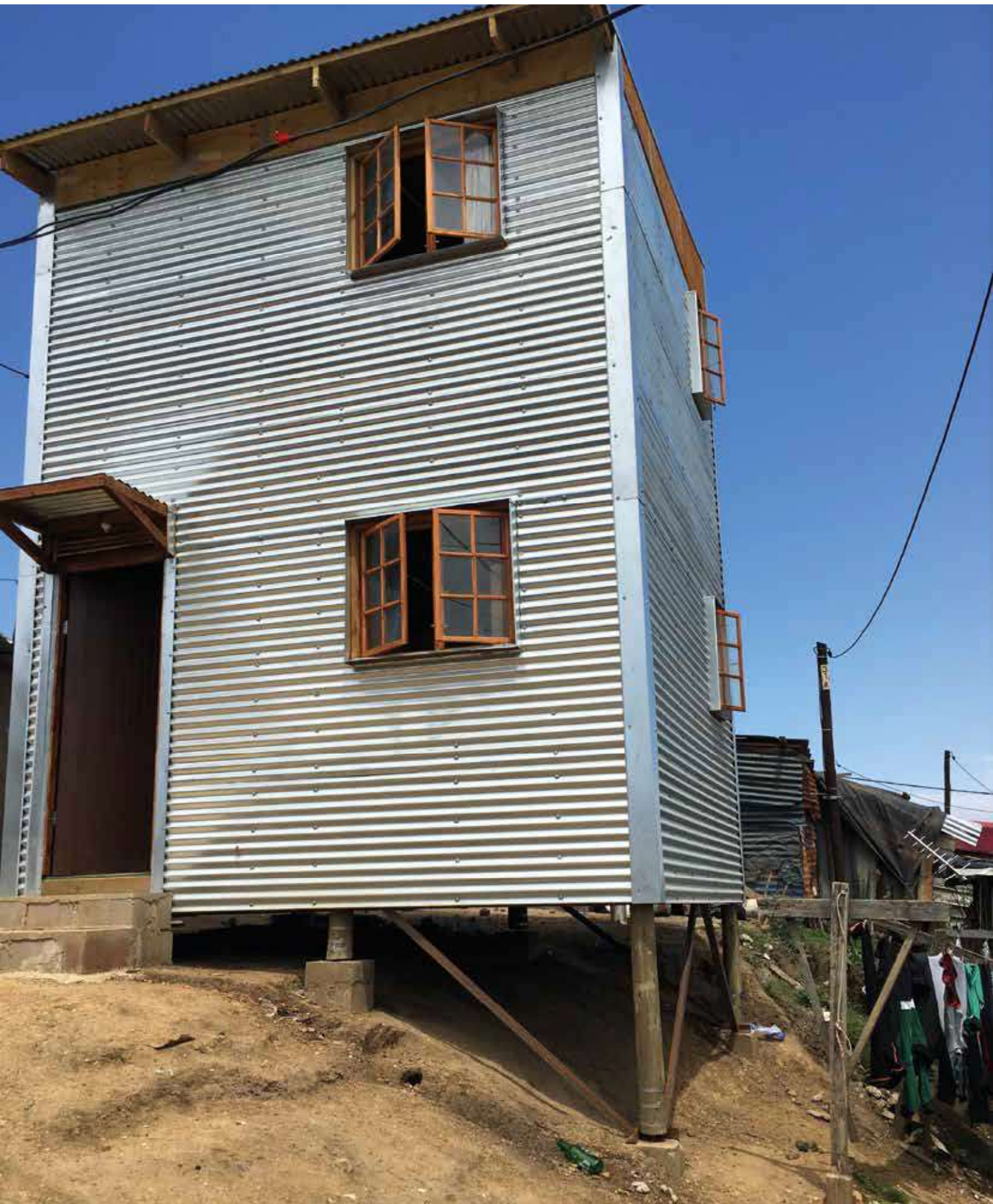
The completed two-storey structure in Parkington informal settlement in eThekweni. Photo: HSRC
