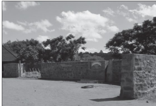
Figure 4: A stone and mortar wall used to form the barrier of the Kgotla (Source: Sebitla, 2018, p. 146)
